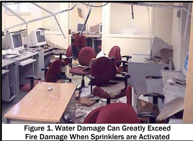
**Figure 1. Water Damage Can Greatly Exceed Fire Damage When Sprinklers are Activated**
